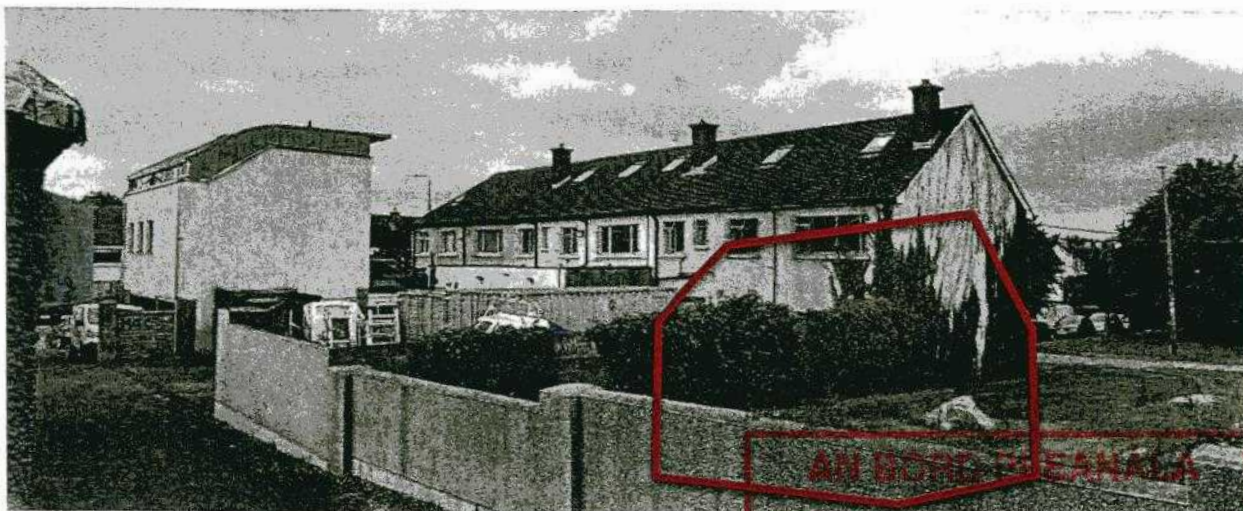
Figure 8.0 Rear elevation of subject site. The contemporary building to the west is noted.
